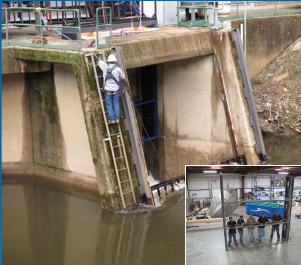
Three-antenna stacked array installed about 10-15 feet downstream of the trash rack location in the Camptonville Diversion Tunnel Intake opening
